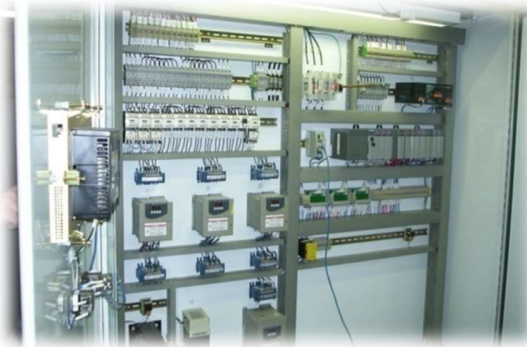
PLC & VFD PANEL
